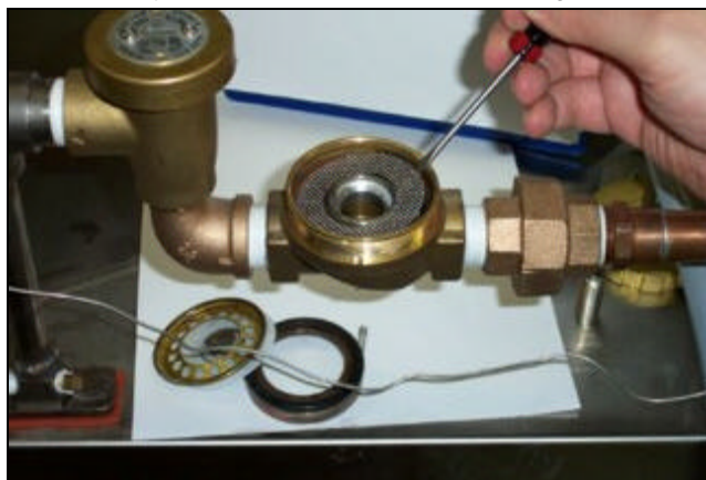
Removing the mesh strainer screen
